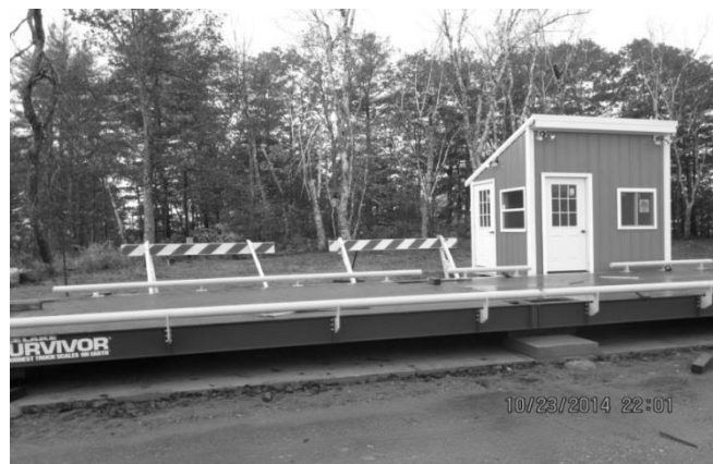
New Transfer Station Scale House
